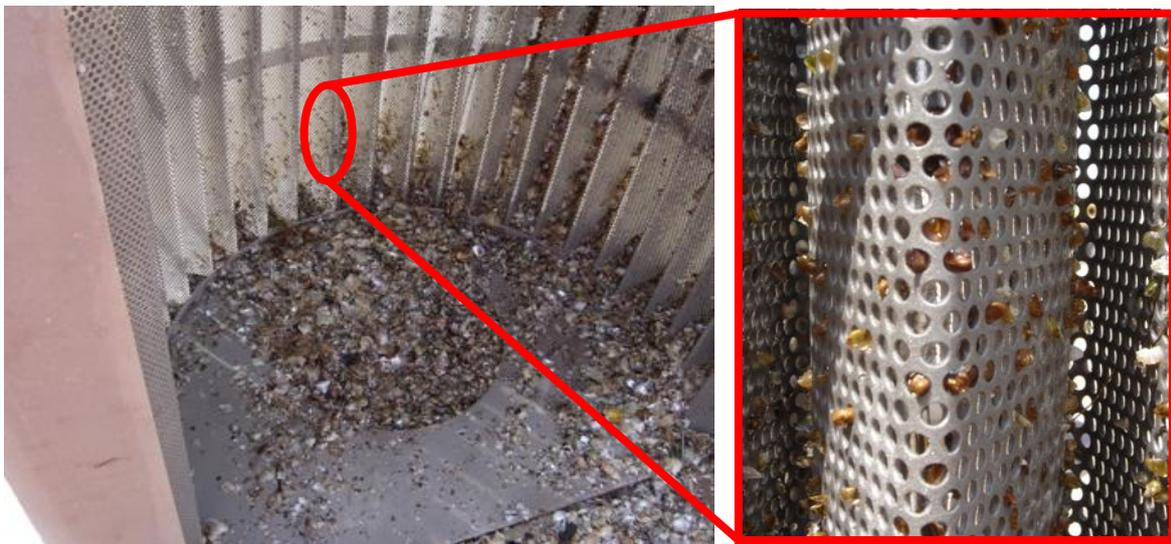
Figure 1 Fouling by oyster shells at a strainer in the year 2007 before P-C was implemented, in front of a heat exchanger at Qatargas
