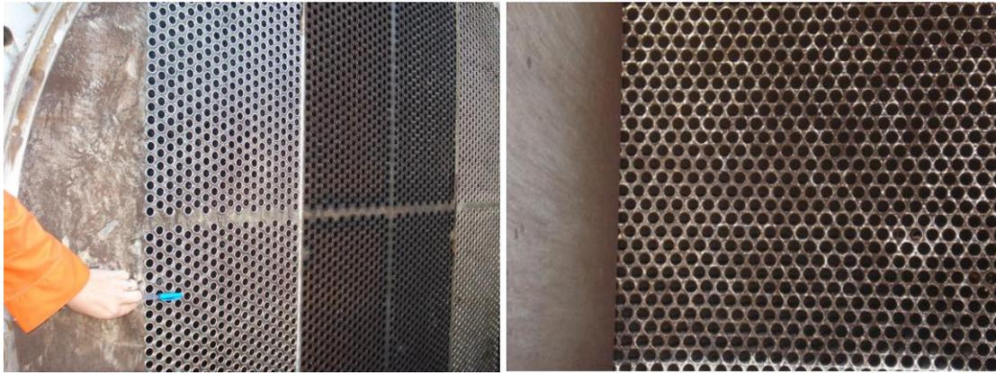
Figure 4 Condenser (left) and Tube (right) endplate after implementation of P-C.
